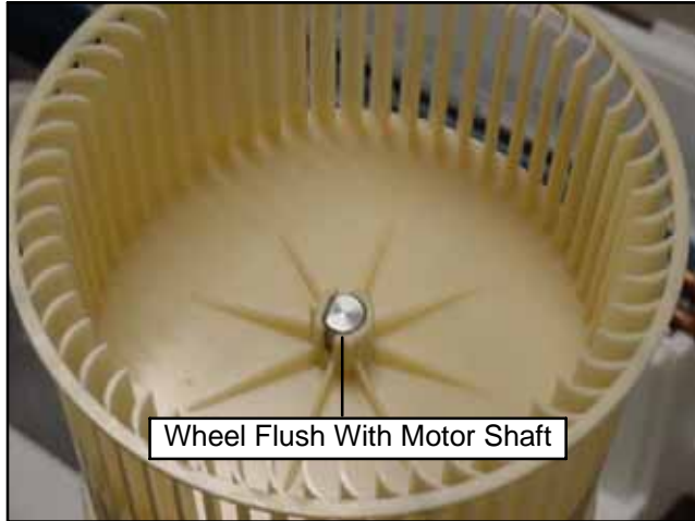
Figure 3-36 Evaporator Blower Wheel (Flush With End Of Motor Shaft)
